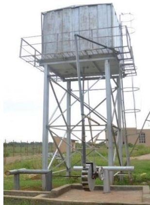
Pumped storage micro hydro power demonstration system and locally fabricated Turbine
