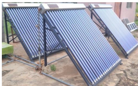
Evacuated tubes forced convection solar water heating system for domestic and industrial applications
