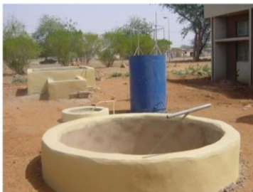
Fixed dome Biogas plant
