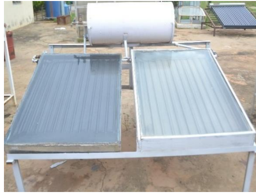
Natural convection (Thermosyphon) Solar thermal water heating systems
