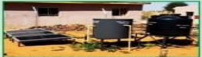
Danjawa 250 litres Solar water Heating System
