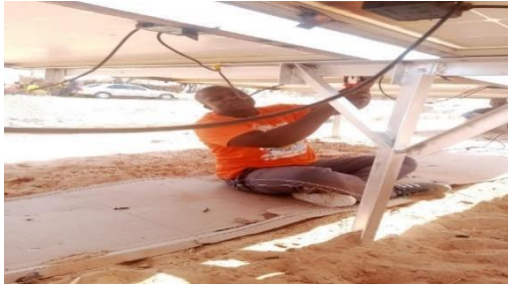
Installations of Solar Modules carried out by SERC Staff in Progress
