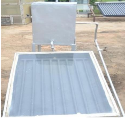
Natural convection (Thermosyphon) Solar thermal water heating systems
