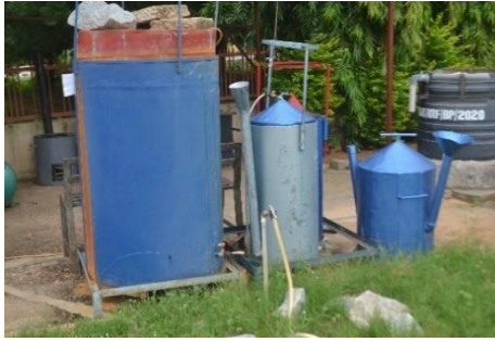
Different biogas plants and gas holders
