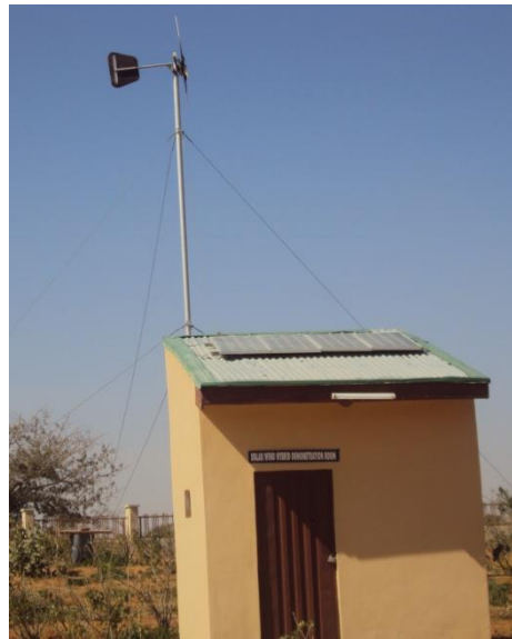
500W Hybrid Wind/Solar Power Constructed by the Centre
