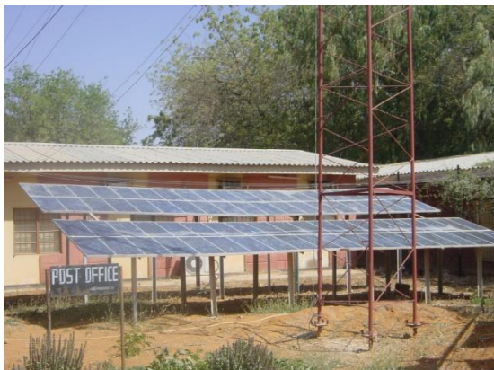
2 Kw Solar PV back – up UDUS Internet System
