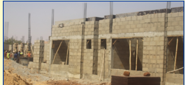
New Senate Building under construction
